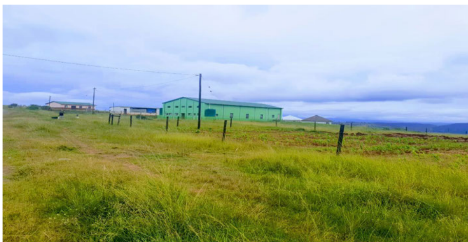
Figure 5.4: The image below is one of the halls that has been built in eMakhuzeni (Springvale)
