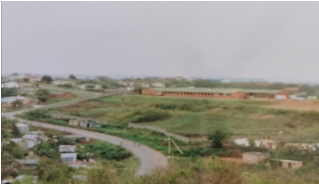
Figure 3.8: A photograph showing a township school building such as the one I attended
