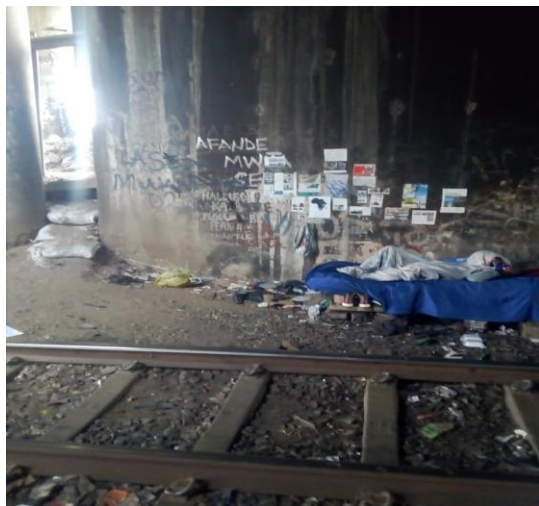
Image 5.4: Under the bridge (Source: San Juan)
