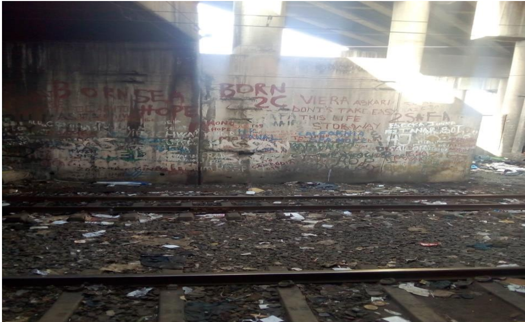
Image 5.3: Railway lines under the bridge (Source: San Juan)
