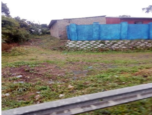
Image 5.6: Safe House (Photos Source: San Juan)
