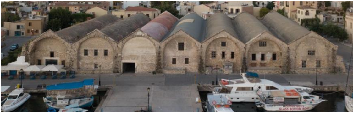
Figure 3- 4: Seven-span shipyard masonry building in Greece, with vaulted roof (Providakis, 2021).
