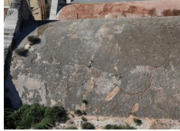
Fig.4b. 6 th vault outside view
