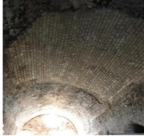
Fig. 4a. 4 th vault – inside view
