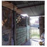
Fig. 5.2.21 Preparation area with grill blocks for ventilation (By Author)
