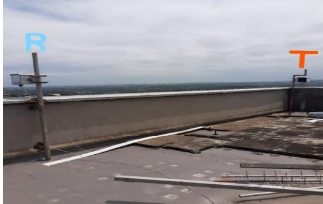
Figure 11: Transceivers Used and the link distance of 7 meters between them
