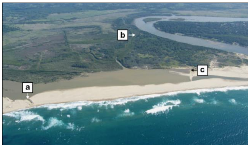
Figure 3-12: Illustration of construction completed in order to transfer water from the Mfolozi River estuary into the St Lucia Lake in 2007. a: Excavation of small channel at a specified overflow level. b: Construction to ensure that the Backchannel could be closed in the case of a flood event level. c: Strengthening the berm at the Mfolozi River mouth to ensure that the berm could not be readily breached by sea water. (Whitfield & Taylor, 2009)
