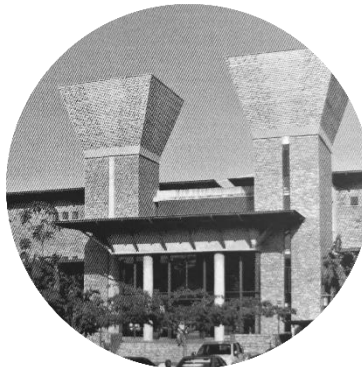
Plate 5.3. 7: Western facade and elements denoting the entrance (Source: Noble, 2011: 47)
