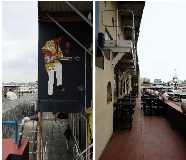
Plate 6.3. 8: The first-floor entrance of the primary facade which contains social space (Source: Author, 2019)
