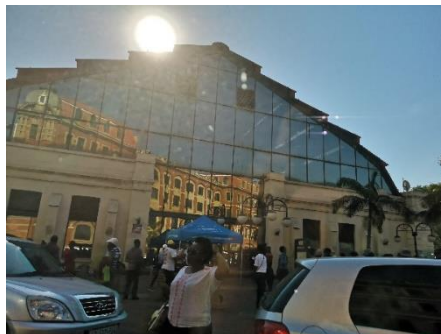
Plate 2.4.1. 2: The Gym on the West side of the site (Source: Author, 2019)
