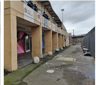
Plate 6.3. 7: The primary facade (Author, 2019)
