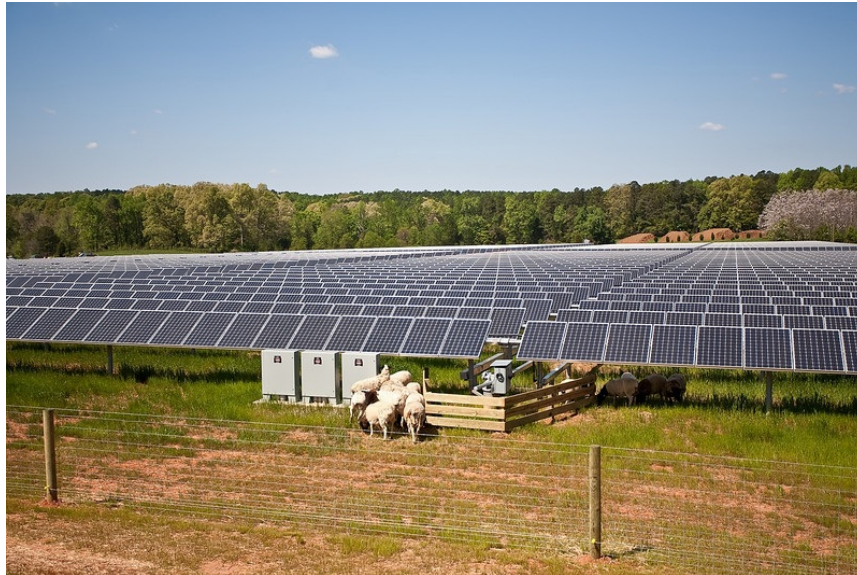
Plate 4.4.3: Solar farm in North Carolina
