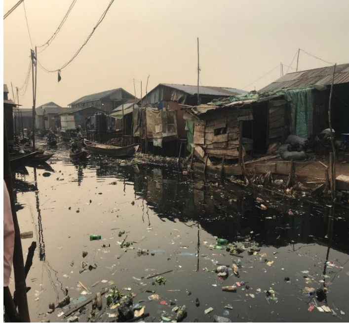
Image 5.1: Informal structures and floating homes along the canal leading to Lagos lagoon in Maroko Area of Lagos city
