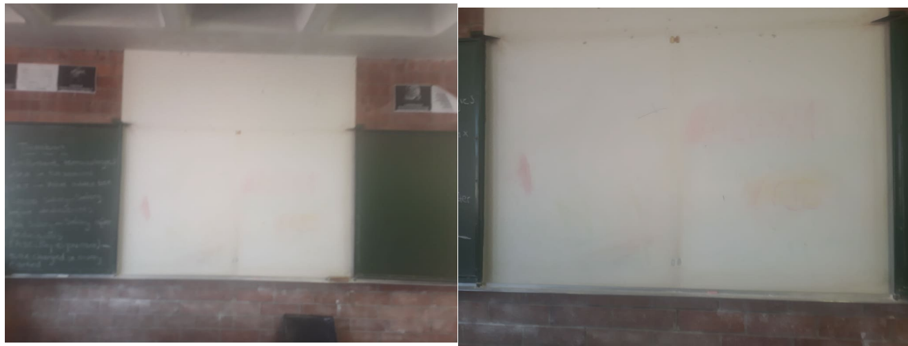
Figure 5.3 The marks on the wall where the projector image was displayed
