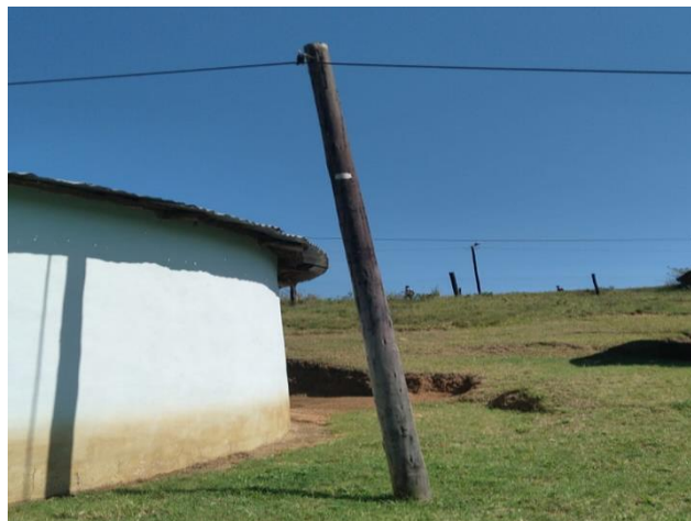
Plate 5.8. Electric cable connected to a homestead in KwaXimba, eThekweni Municipality, KZN
