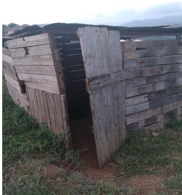
Plate 5.7. Traditional pit latrine or pit toilet built by household members in KwaXimba, eThekweni Municipality, KZN
