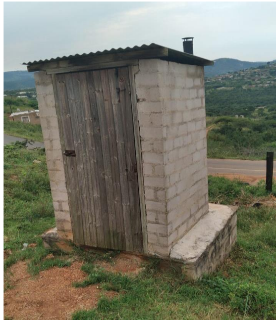
Plate 5.6 Slab pit latrine or pit toilets in KwaXimba constructed by the eThekweni Municipality, KZN
