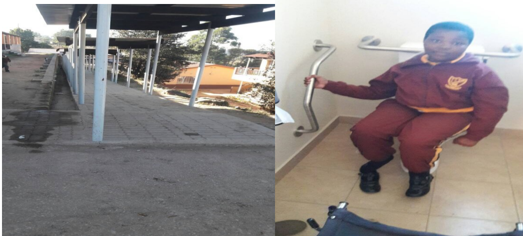
Figure 17- Examples of some improvements made in the school infrastructure as part of the implementation of inclusive education.
