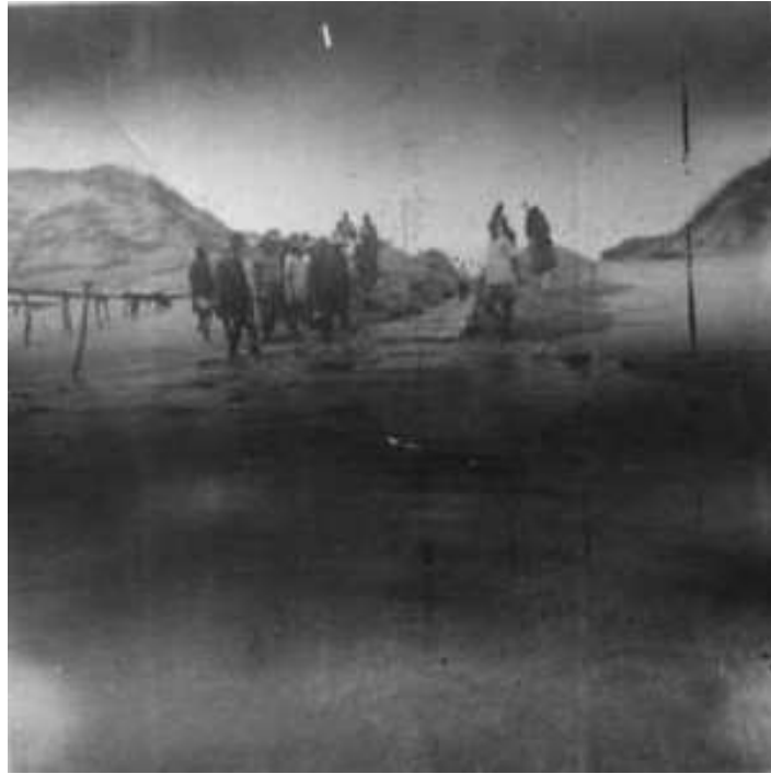
Plate (a): Labourers moving sand from the banks of the Umfolozi River to divert its course into the Indian Ocean, 1952 (Photo supplied by Nidia Brits)
