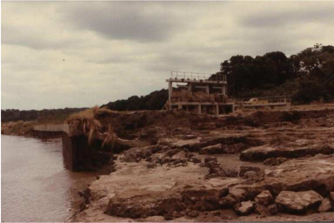
Plate (i). Cyclone Demoina damage to the bank between the Umfolozi River and Link canal at the Intake Works, February 1984 (Photo supplied by Nidia Brits)
