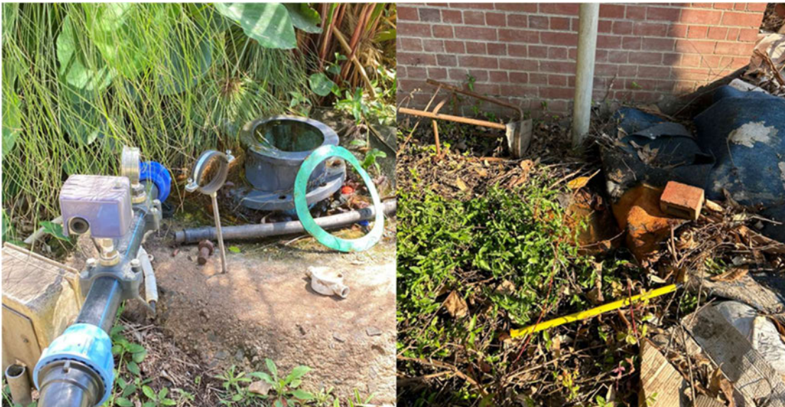
Figure 5.3 Freely flowing boreholes in Pietermaritzburg and Durban
