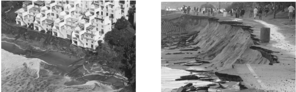
Figure 1.1. 2007 Storm damage to (a) Ballito Bay and (b) Umkomaas (Mather, 2012)
