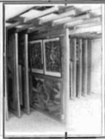
ILL. 103: Sliding rack system which is used in the paint store at the conservation facility. Ref. Author
