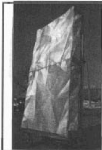
ILL. 63: A single crumpled aluminium mesh panel before installation into the building envelope. Ref: http://www.walkerart.org/index.wac
