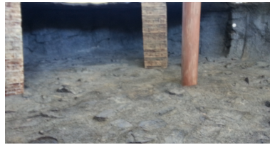
Figure 3.8: Picture of pillars taken from the artificial underground mine
