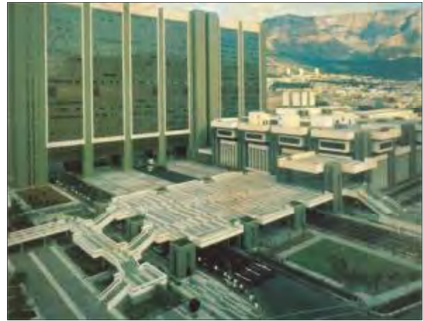
Plate 46: Pedestrian bridge piazza links Civic Centre to Opera House (Wale, 1979: 1)
