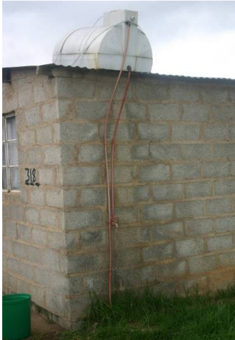
Figure 7: Water supply tap connected behind one of the houses, far removed from the front door. (Photograph by: Siyabonga Zondi)
