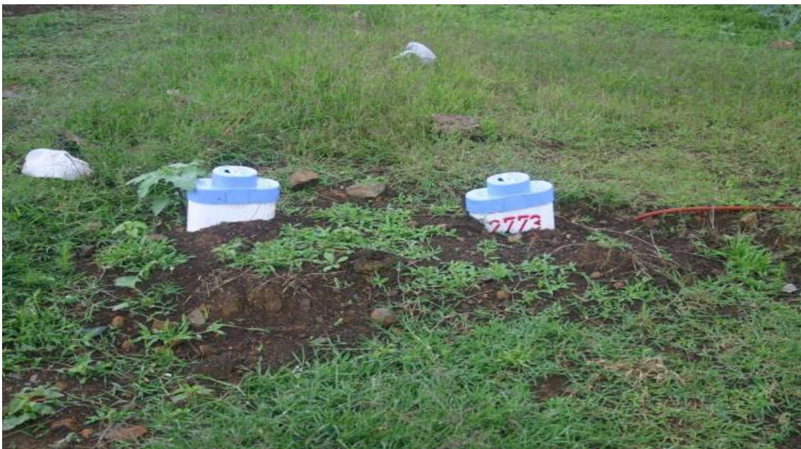
Figure 8: Water reticulation network that was shared by more than one household. Water meters were susceptible to vandalism and tampering which may affect water supply. (Photograph by: Siyabonga Zondi)
