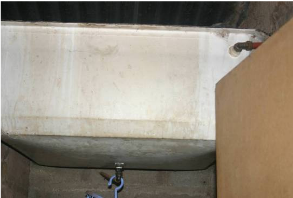
Figure 3 b: Indoor low-pressure tank mounted above the toilet seat. (Photograph by: Siyabonga Zondi)
