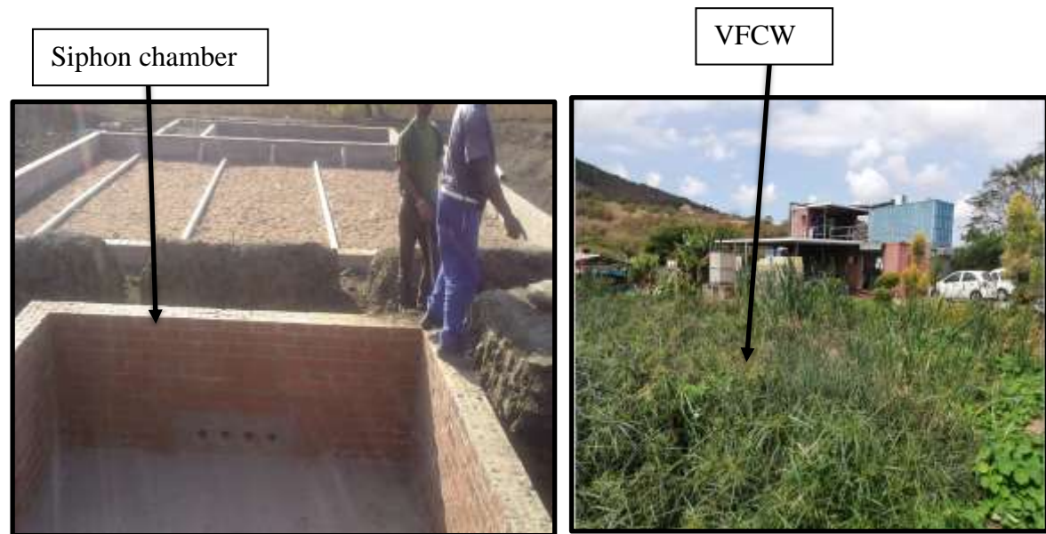
Figure 18: Left - Siphon chamber and VFCW during construction at NLM DEWATS. Right – Plant material at NLM in June 2019.
