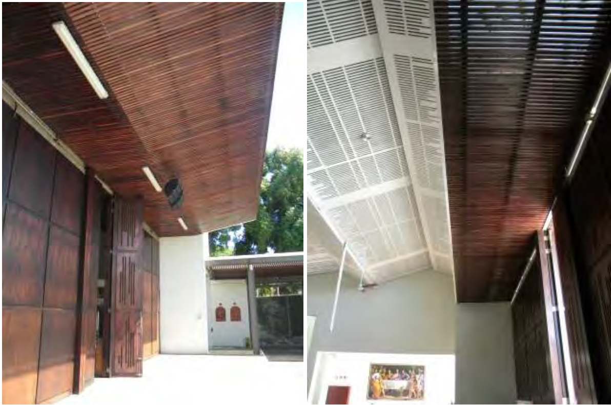
Fig 4.26 Large timber doors and panelling. Source: Author, 2014. & Fig 4.27 Timber panelling within the nave. Source: Author, 2014.
