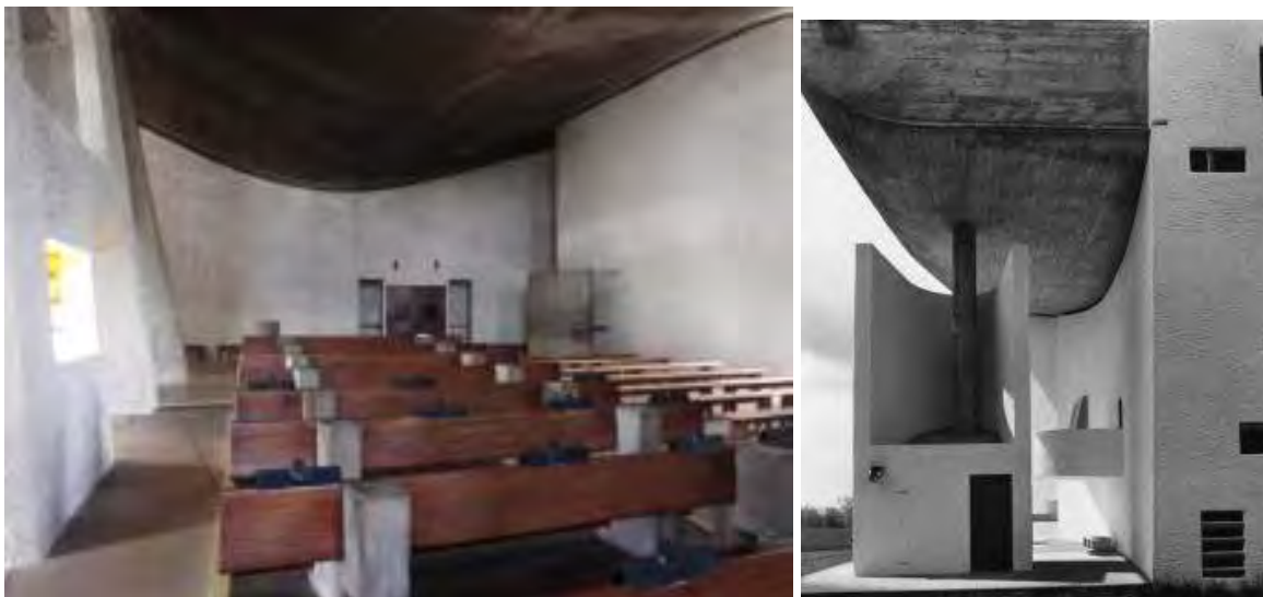
Fig 3.9 Timber and cast concrete benches in chapel. Source: http://www.architectureis.org/2012/07/27/a-long-journey-6/ , Online (Accessed on 29 April 2014) & Fig 3.10 North façade showing side of outdoor sanctuary. Source: http://www.artandarchitecture.org.uk/images/conway/01eedc15.html , Online (Accessed on 29 April 2014)
