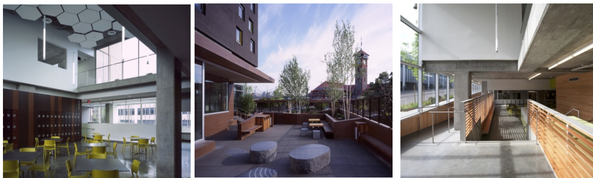
Figure 4.10, 4.11 & 4.12: From left, space for lockers and dining, secure outdoor socializing space and the entrance into the day shelter. All show the multi- pronged approach that reaches beyond the necessary and into nurturing. ( http://www.dwell.com )
