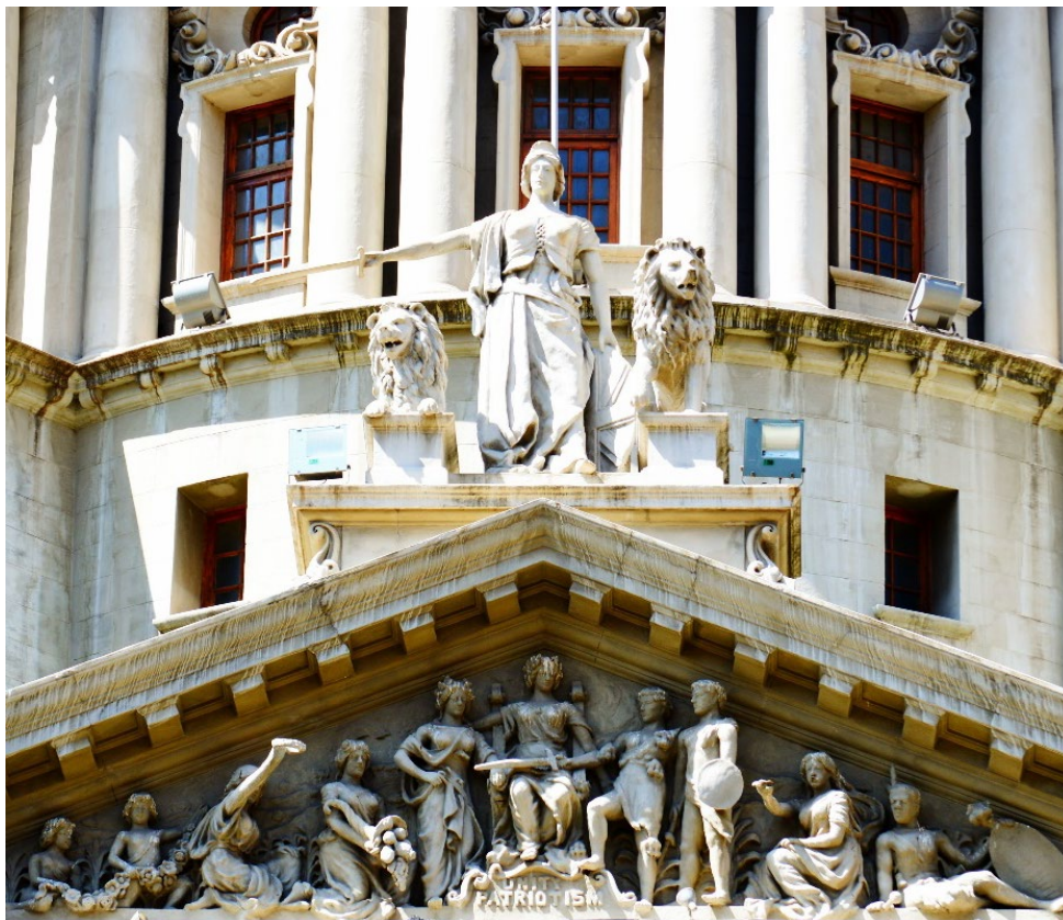
Fig 1.3. The architecture sculpture at the front of Durban City Hall, showcasing pan-European motifs, taste, and symbolism.
