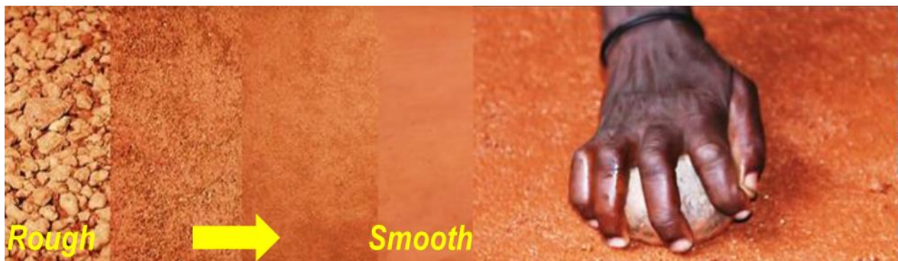
Figure 8.2b: illustrates the floor construction technique in one of Francis Kere projects whereby women learn through repetition of the same thing. They first get it wrong; redo and it improves till when the surface is smooth. Source: Modified by the Author from https://www.designboom.com .
