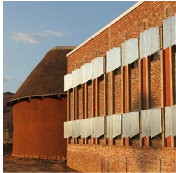
Figure 4.2f: illustrating Solar devices to achieve a suitable IEQ at Seven Fountain. (Source: www.eastcoastarchitects.co.za/ )
