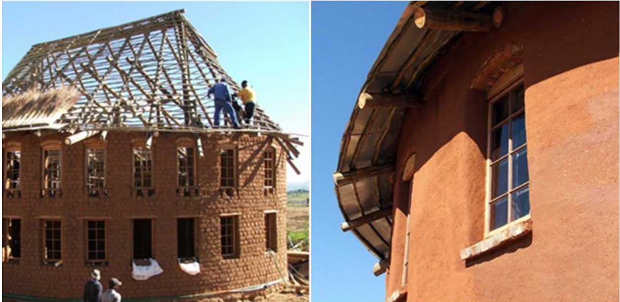
Figure 4. 2a illustrating adobe earth as abundant and renewable materials used in multipurpose building, Seven Fountain School in Kokstad. (Source: https://www.designindaba.com/ )
