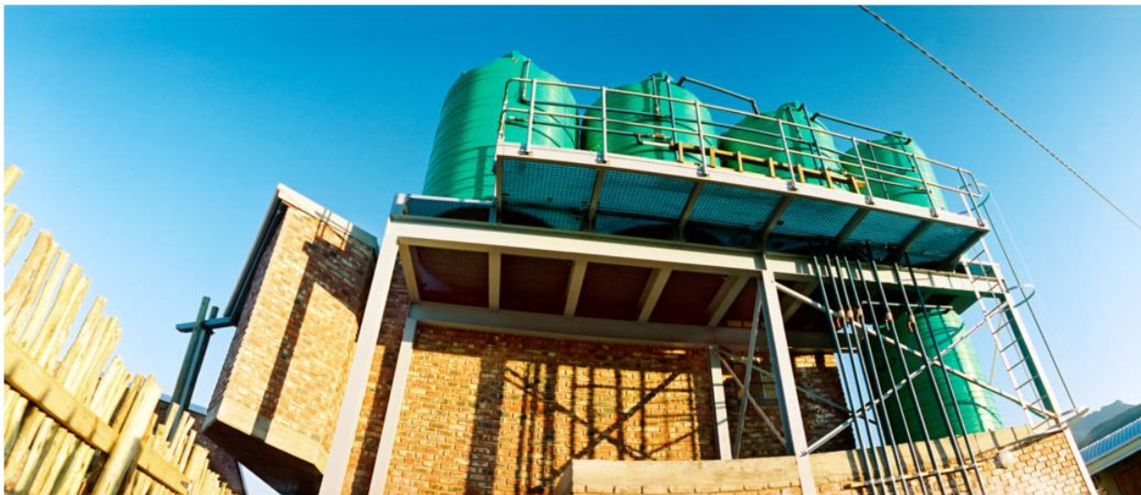
Figure 4.2c illustrating rainwater tanks to collect all rainwater from impermeable surfaces and used to flush toilets and water vegetables which is in line with protecting the natural environment principal. (Source: http://www.angelabucklandphotography.com/ )
