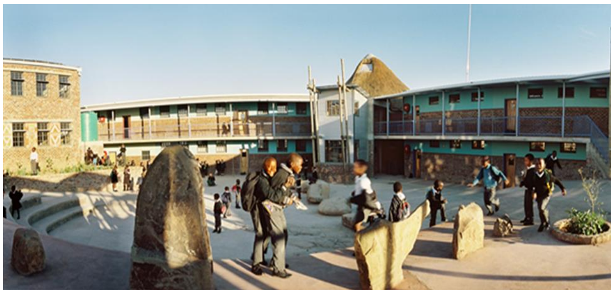
Figure 4.2e: illustrating children playing in a gathering & performance space facing North orientation and classrooms with covered walkways as solar devices to ensure space gets natural light and warm in winter. ( Source: https://www.eastcoastarchitects.co.za/ )
