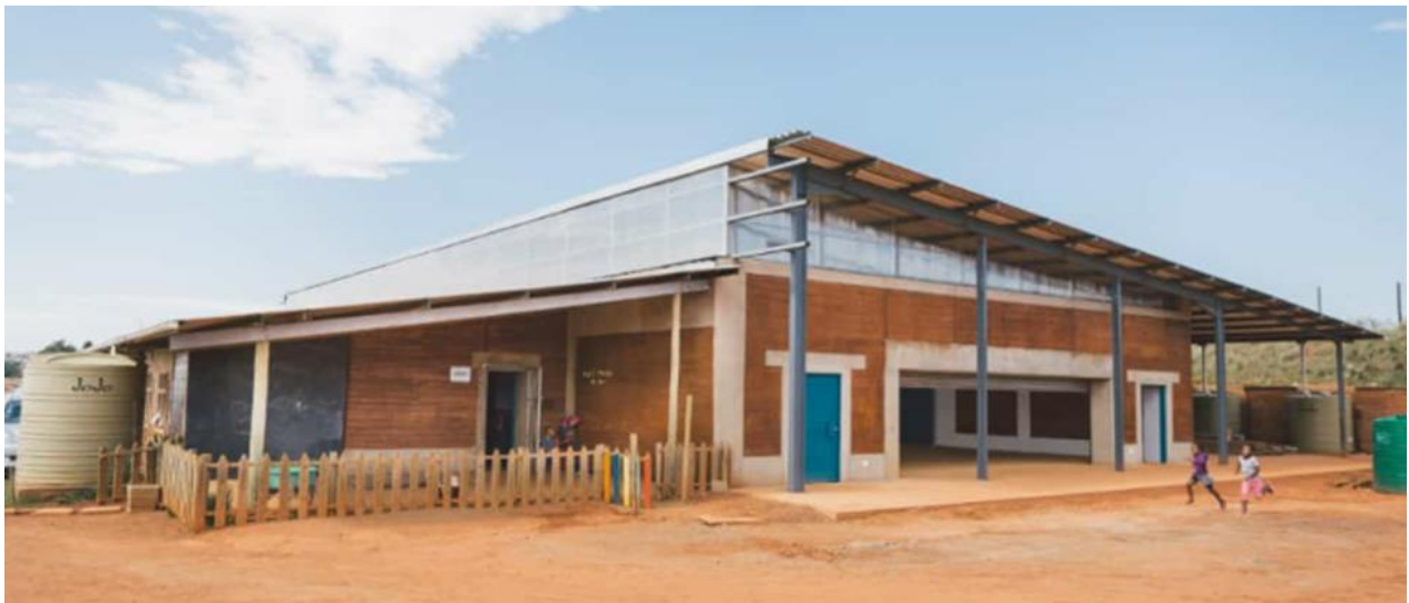
Figure 6.2a: illustrates the exterior of IthembalamaMpumuza ECD. Source: (by Author, 2019)
