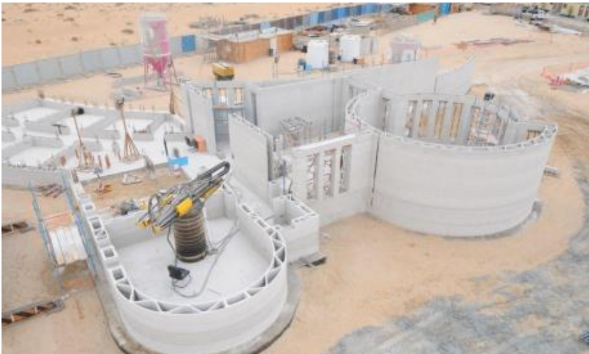
Figure 1.25. Largest 3D Printed Building in the World, Dubai (www.engins.org)
