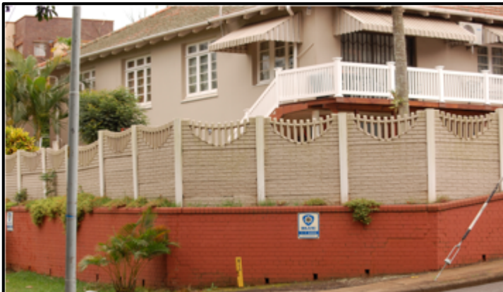
Figure 12: A home with a low brick wall and a precast fence above it. It appears that this was done in stages as the owner became more crime conscious, possibly experienced crime or simply made these additions as a result of fear of crime.
