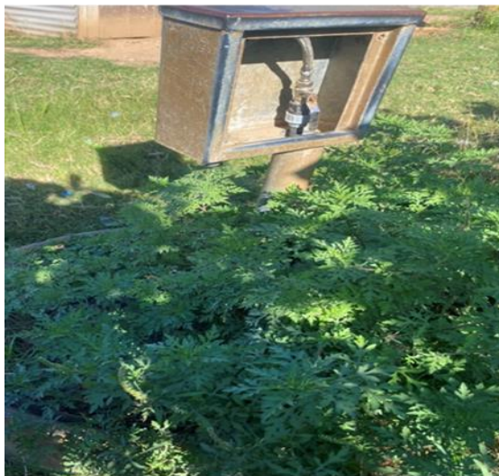
Plate 5.9 A dysfunctional standpipe within the Mkhukhuze community
