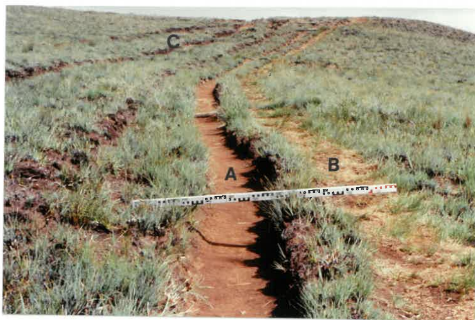
Figure 3.6 Multiple footpaths on the Bannerman Hut approach path (A indicates the primary path with water breaks installed on it, B indicates a newly forming secondary path and C indicates additional secondary paths)
