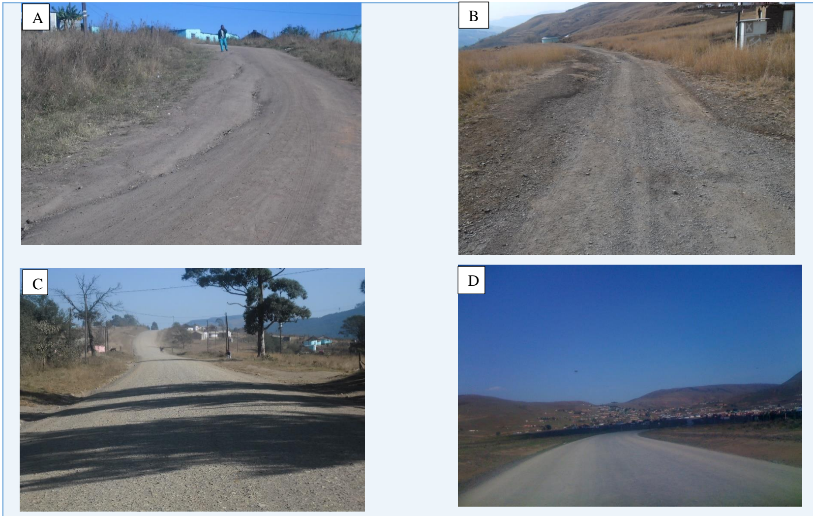
Figure 5.3: Figure 3: The variation of road surface conditions in some of the road lengths selected for this study. The surface road conditions were: (A) very poor (B) poor (C) good and (D) excellent.
