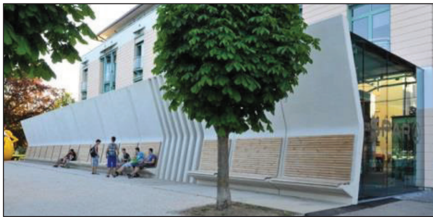
Fig 4.3.1 Spar Gmunde, grocery store exterior with integrated street furniture
