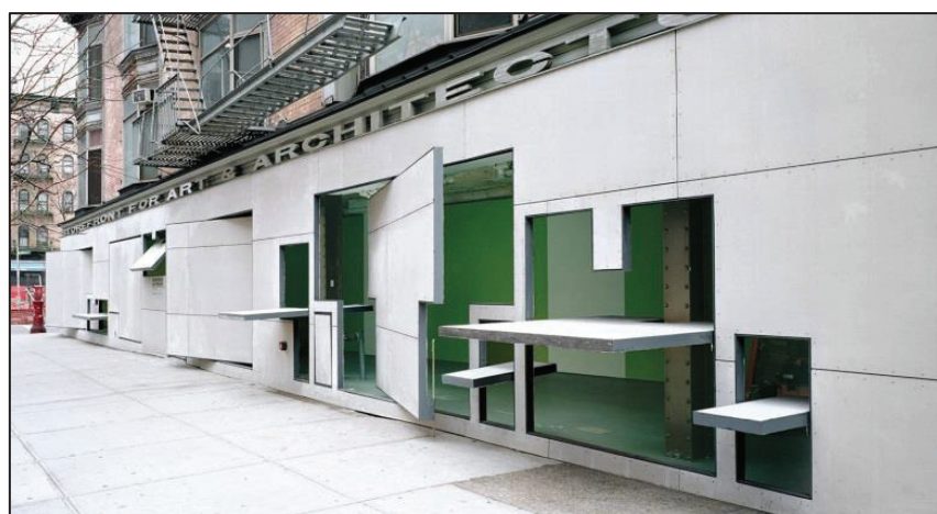
Fig 4.3.2 Store front gallery facade challenges the distinction between public & private space.
