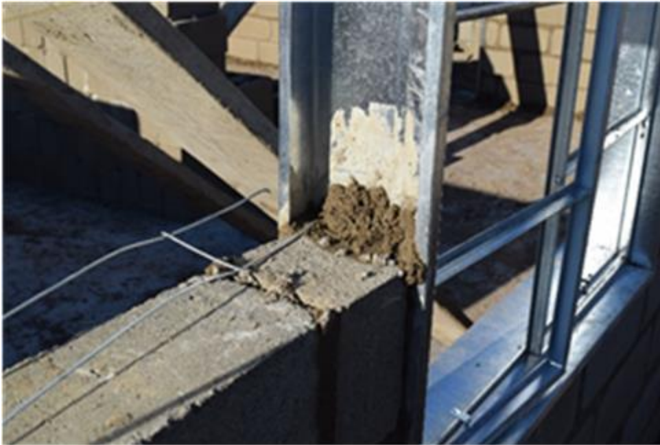
FIGURE 31. BLOCKS FIT INTO FRAMES AND GAPS FILLED WITH MORTAR (SMITH 2019)
