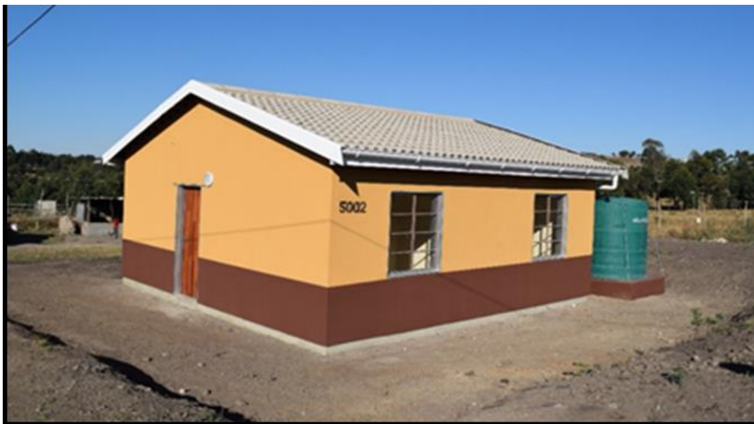
FIGURE 13. RDP HOUSE IZINGOLWENI 2016 (SMITH 2015)
