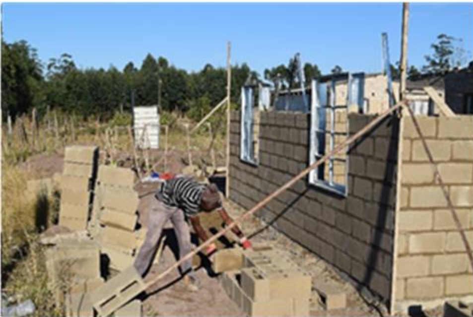
FIGURE 30. WALLS BUILT WITH WHOLE BLOCKS (SMITH 2019)
