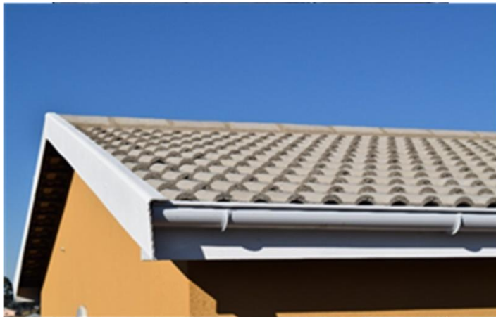
FIGURE 35. CEMENT TILE ROOF, PLASTIC GUTTERING ON FACIA BOARDS (SMITH 2019)
