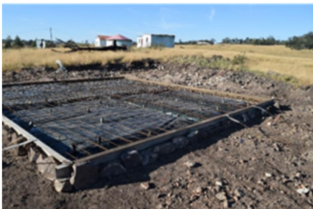
FIGURE 28. STONES ARE USED TO FILL GAPS AROUND THE SHUTTERING (SMITH 2019)
