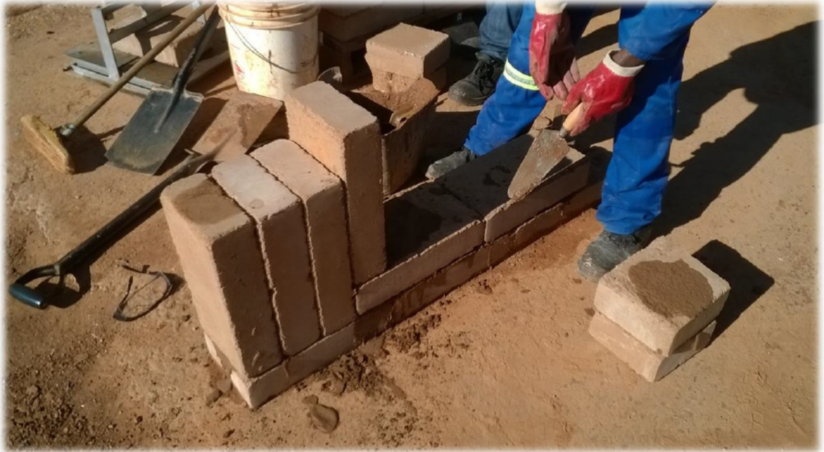
Building demonstration – compressed soil blocks laid together using cement/soil slurry
