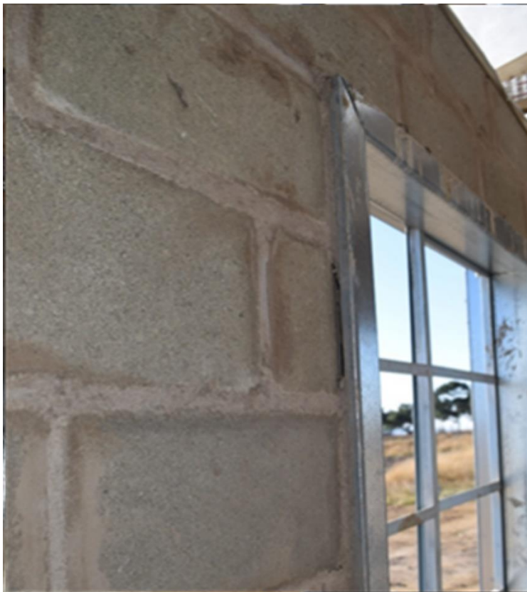
FIGURE 34. THE PLASTER IS APPLIED FLUSH WITH WINDOW-FRAME (SMITH 2019)
