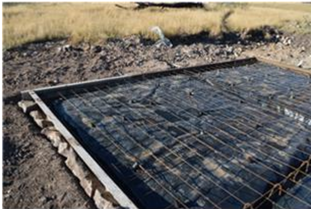
FIGURE 26. FOUNDATIONS MADE WITH SHUTTERING (SMITH 2019)
