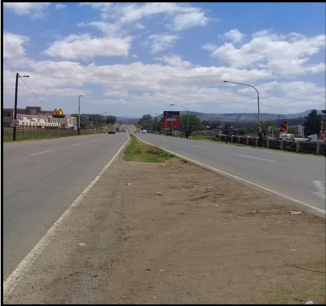
Plate 5.5: Greater Edendale Mall along the Edendale Corridor
