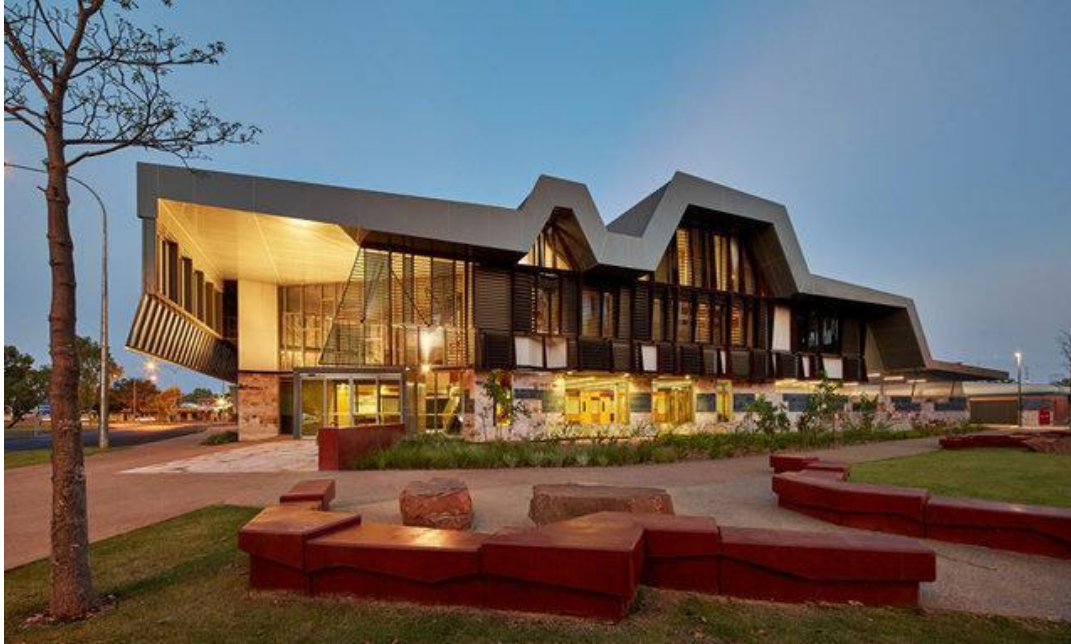
Figure 18: The Outdoor Waiting Area Kununurra Courthouse Complex
