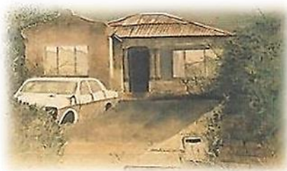
Figure 12 Typical improvements-not an uncommon sight to see a car parked in the yard
