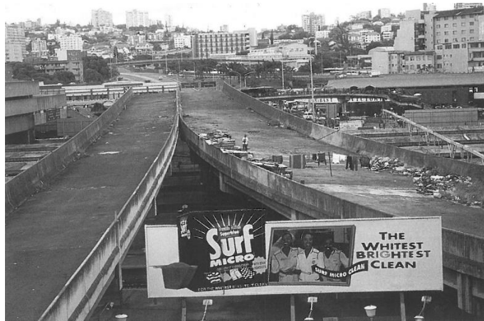
Figure 84: Before -The incomplete and unused vehicular flyovers. (Source: KZ-NIA Journal 3, 2001)
