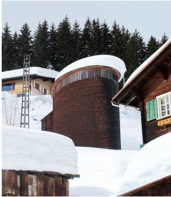
Figure 62: The chapel, close to the local traditional houses, is erected with wooden shingles and snips. The roof of the chapel resembles a boat's hull. An elegant, minimal solution is to mediate between the expressive roof and the more conventional wooden base below: a ring of vertical wood columns and glass panels crowning the chapel that allow the interior space to be penetrated by natural light. (Source: Kalvelage, 2016)
