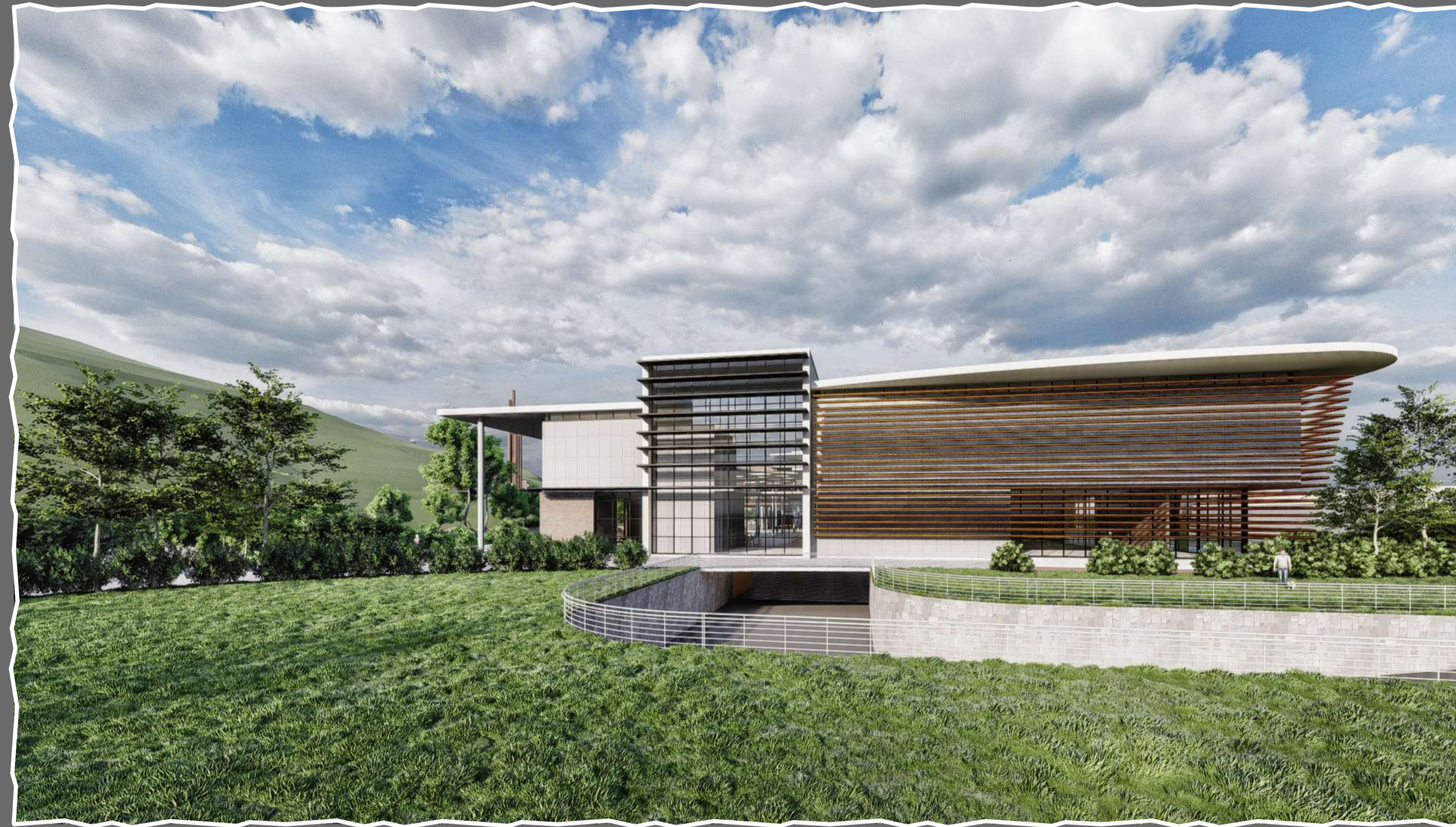
Entrance to Basement Parking
