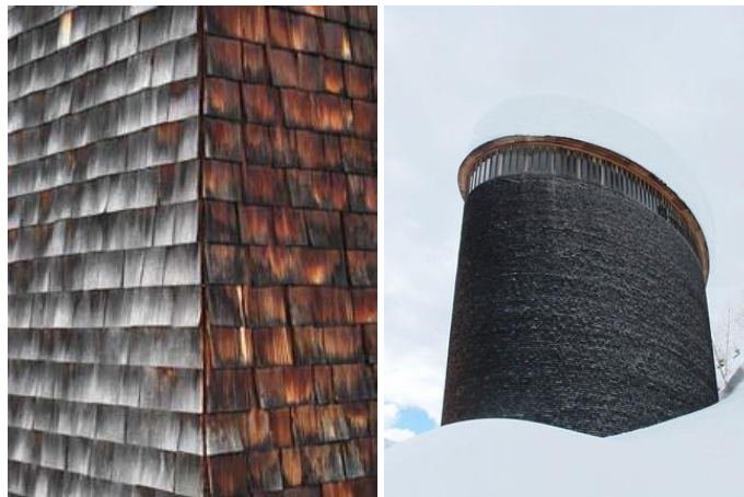
Figure 63: The material is baked wood with brownish red colour. The timber on the south facade remains its original colour. The colour of its edge got changed under different sunlight exposure. The north facade turns into a grey colour since it's always covered with steam. The trace of time and nature is the exclusive decoration of the facade. The shadow of the entrance, the trace of the waterdrop, the sunlight, the rainfall, the snowfall, all of them are documented on the facade. (Source: Kalvelage, 2016)
