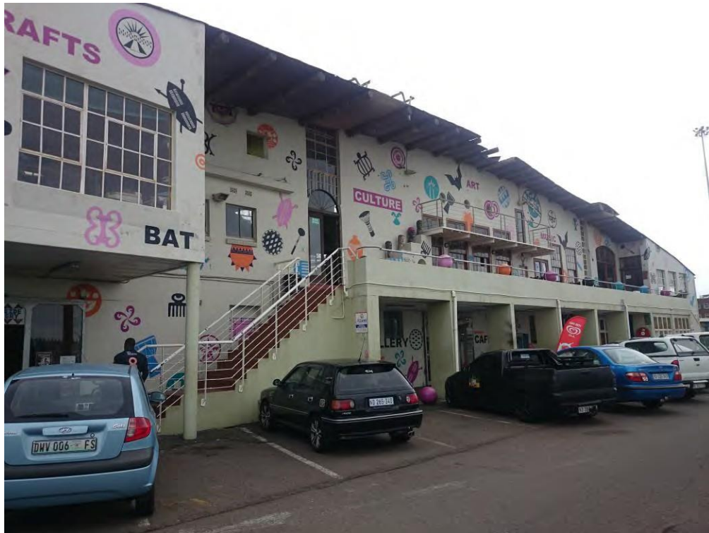
Figure 86: Harbour facing elevation of the BAT Centre. (Source: Naidoo, 2014)
