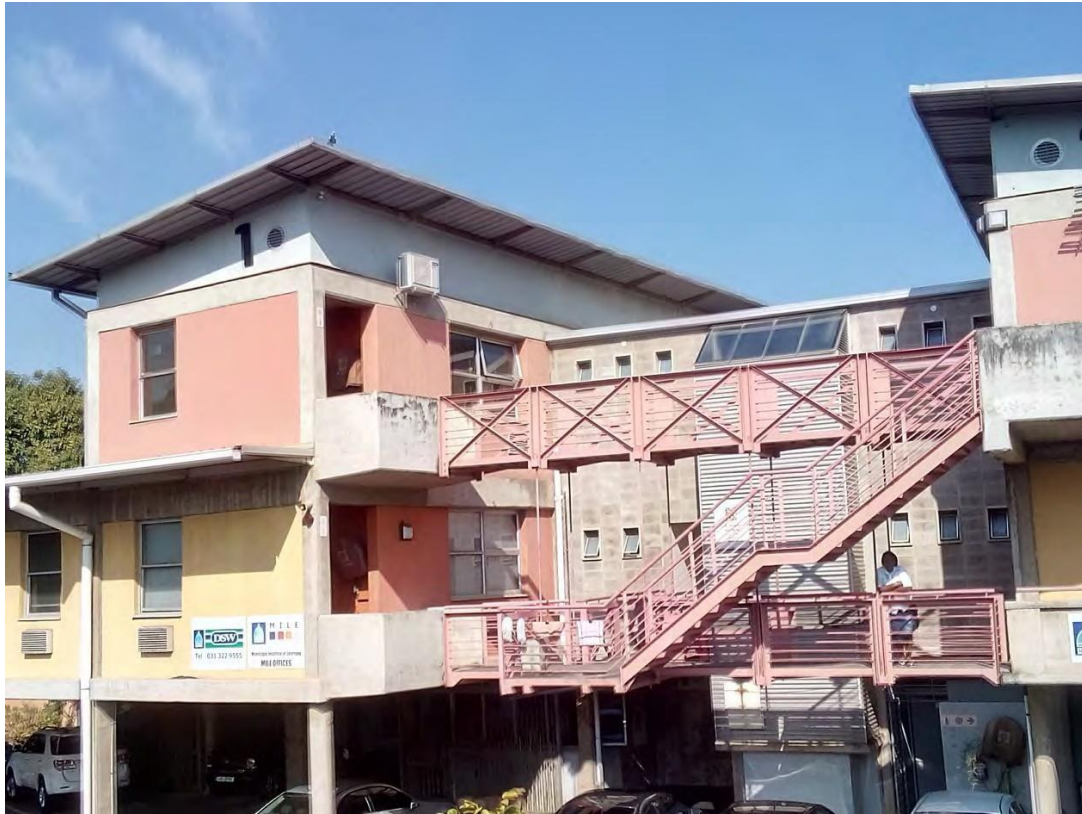
Figure 106: The exposed concrete superstructure with infill block work, the different colours and various materials together with an interesting building form highlights important aspects of critical regionalism. (Source: Pillay, 2014)
