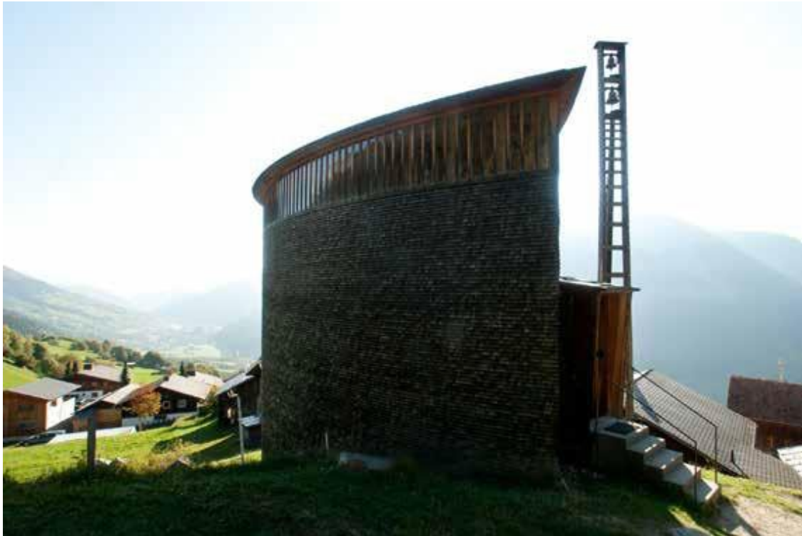
Figure 58: This Chapel is a modest wooden building situated on a mountain slope. (Source: Kalvelage, 2016)
