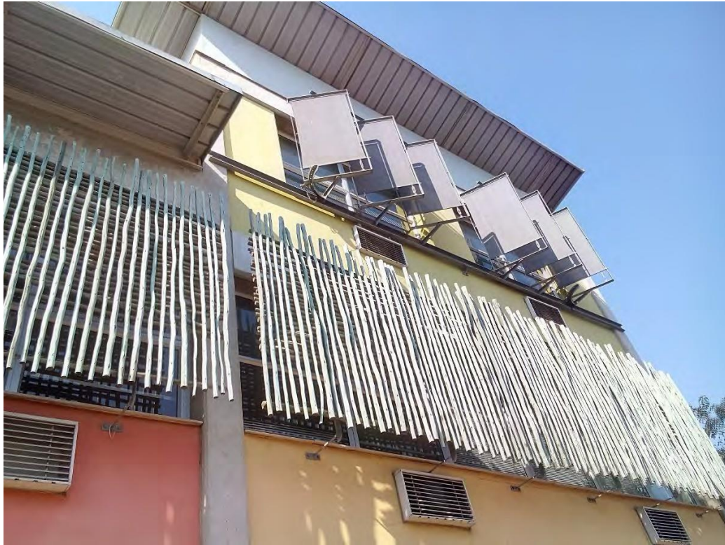
Figure 105: Different types of sun screen devices used on the west elevation. (Source: Pillay, 2014)
