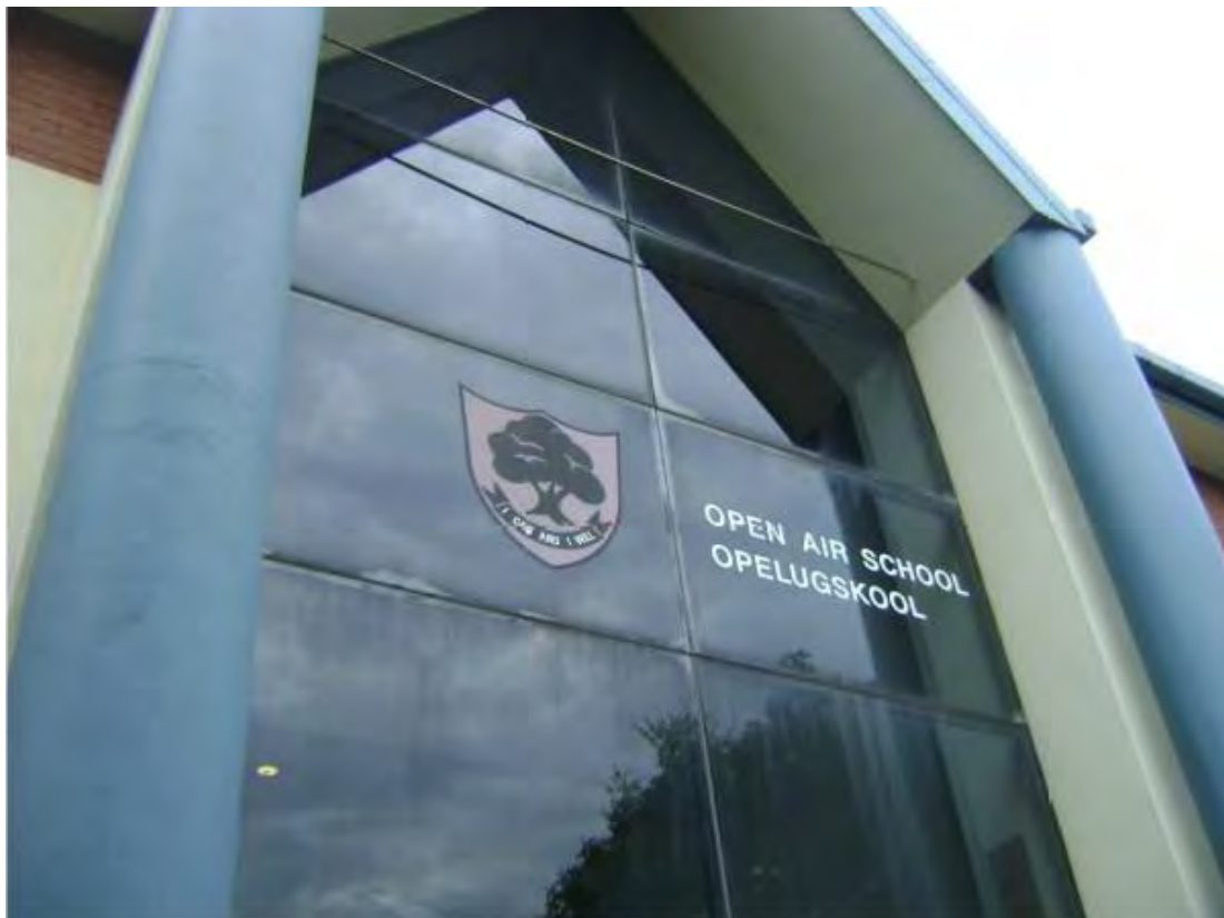
Figure 30: Entrance canopy and glass façade
