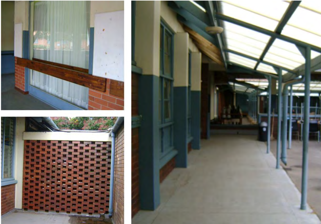
Figure 32: Photos of corridors (textures/bris-soleil)
