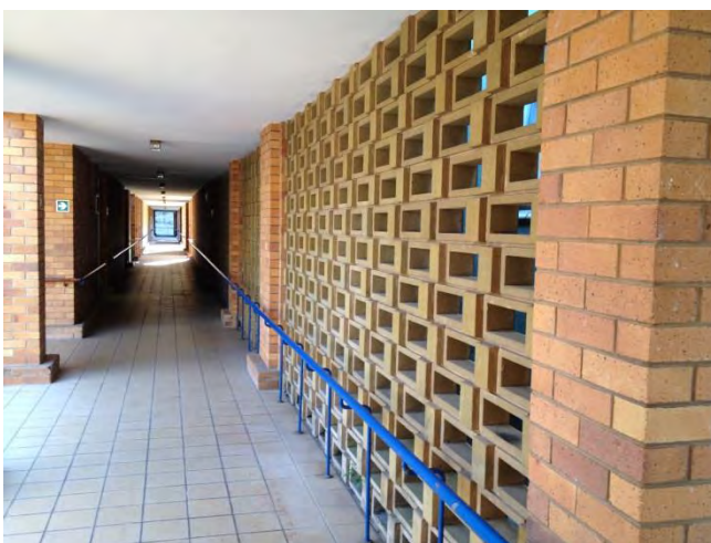
Figure 21: Brise-soleil along corridor
