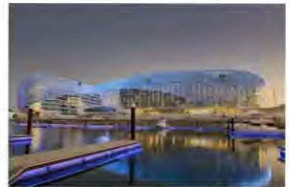
Fig 3.2.1.5 Covering membrane of the Yas Marina
