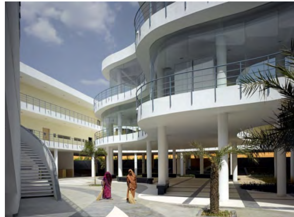
Figure 4.2.2.3: Curving courtyard walls
