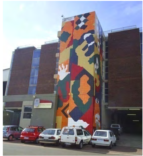
Figure 5.2.2.1: Front view of school
