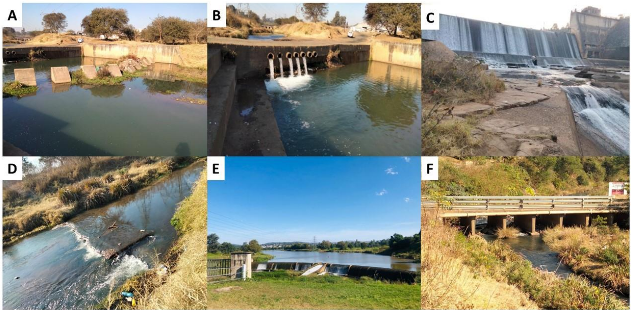
Figure 3.2: Examples of different barriers observed, where (A) is a canal, (B) a culvert, (C) a dam, (D) a ford, (E) a weir and (F) other in the assessed waterways in Pietermaritzburg, South Africa.
