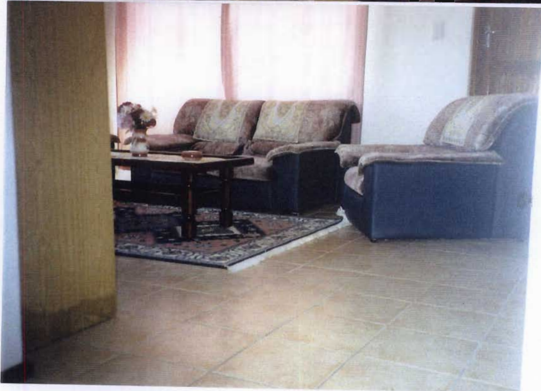
Figure 10c. N.B. Use of ceramic tiles in the place of wall-to-wall carpet.
