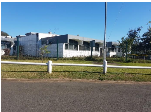
Figure 57 Image showing building form from road (By author, 2018)
