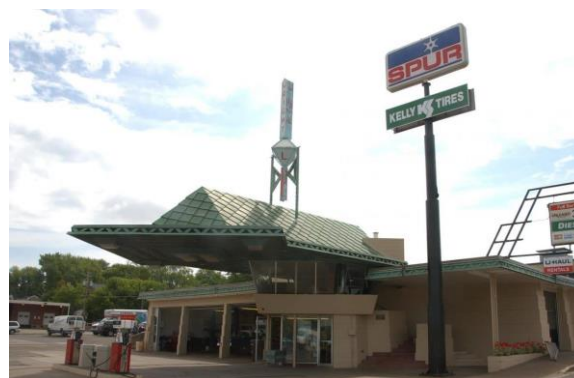
Figure 2 Image showing Lindholm service station ( https://franklloydwright.org/site/lindholm-oil-company-service-station/ )
