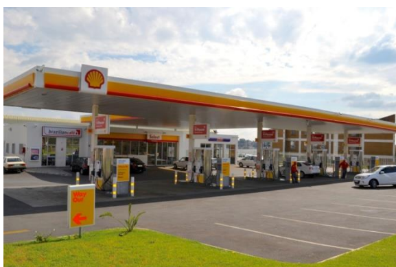
Figure 3 Image showing the evolution of the fuel station ( http://www.2oceansvibe.com/2016/04/25/watch-shell-garage-employees-kick-the-crap-out-of-this-guy-video/ )
