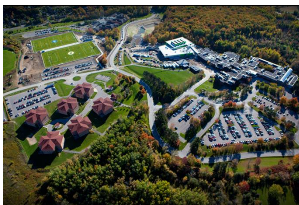
Figure 38 Aerial Image showing context of Kawartha Trade Centre ( https://www.archdaily.com/800181/sir-sanford-fleming-college-kawartha-trades-and-technology-centre-perkins-plus-will )
