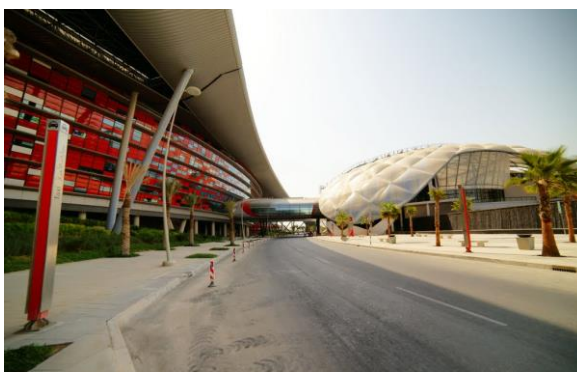
Figure 35 Roadside elevation of façade
