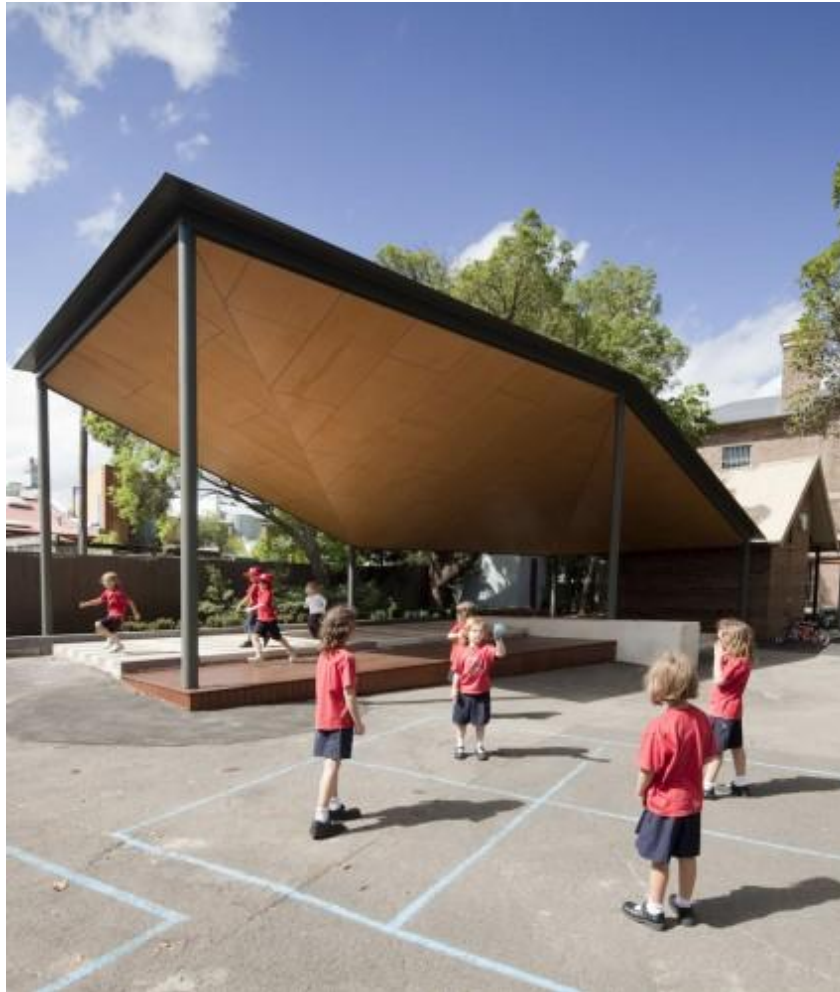
Plate 3.49. (Web 11) An outdoor communal gathering space that can be used for a variety of functions
