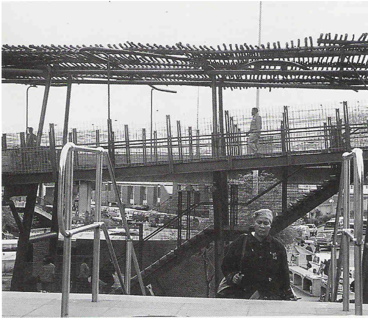
Plate 4.7. (Dobson, 2001: 10) Market Road Bridge
