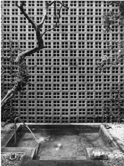
Plate 28: ( ungovernable.tumblr.com ) Use of airbrick screen walls
