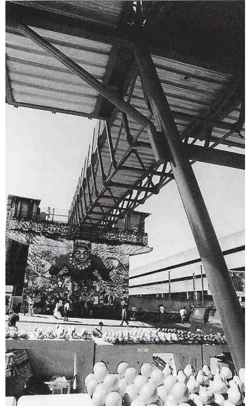
Plate 10: (Dobson, 2001) Market Road Bridge
