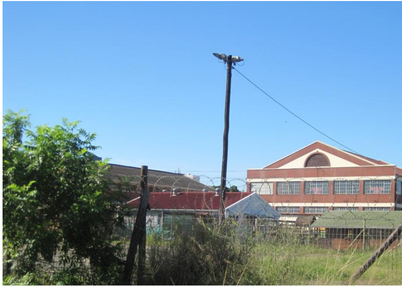
Plate 22: (Author) View of the MMD building from the North
