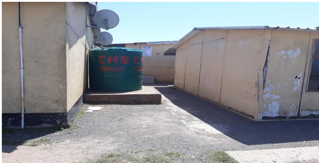
Figure 16: Satellite dishes for DSTV and the internet connection at School C
