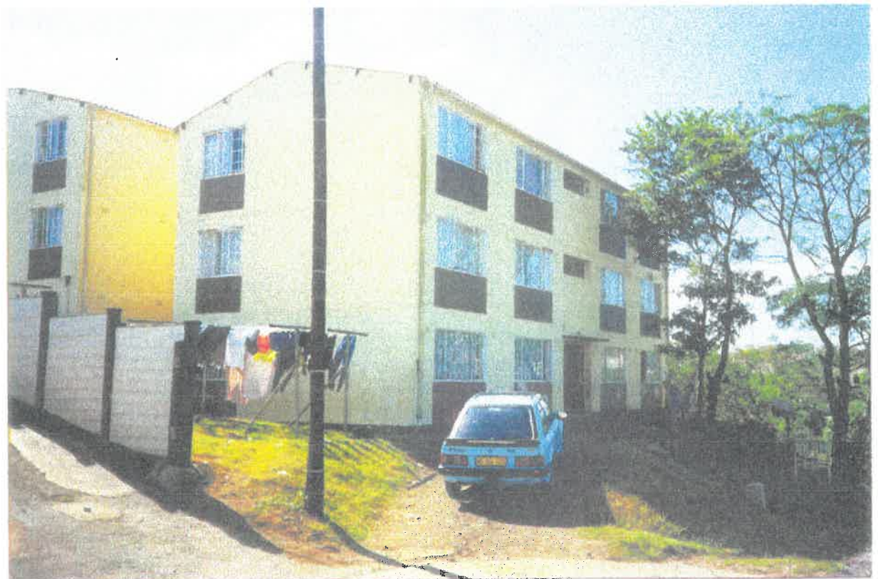
9. Inadequate space for parking and children to play.
