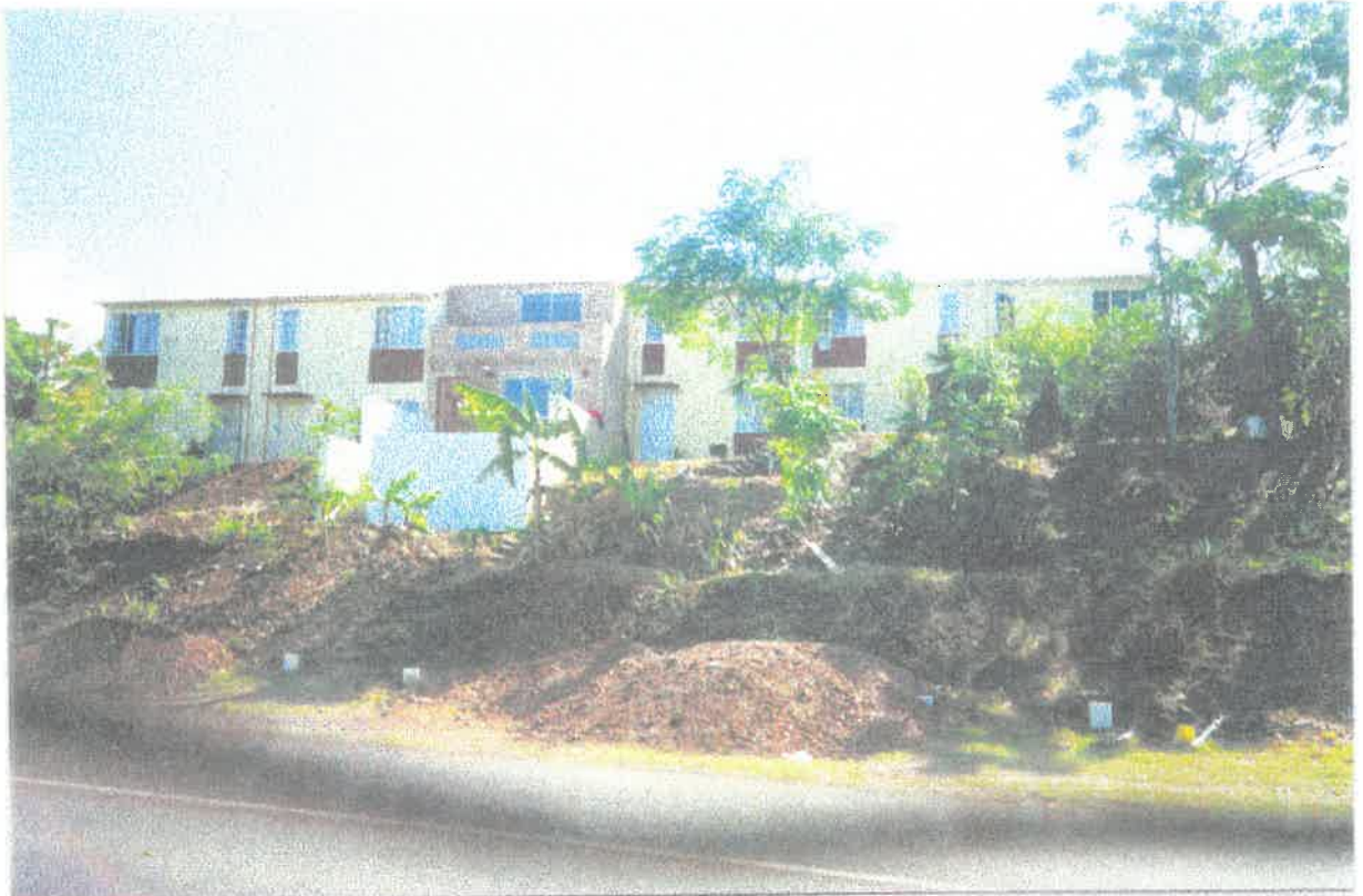
10. Extension to recently purchased duplexes.
