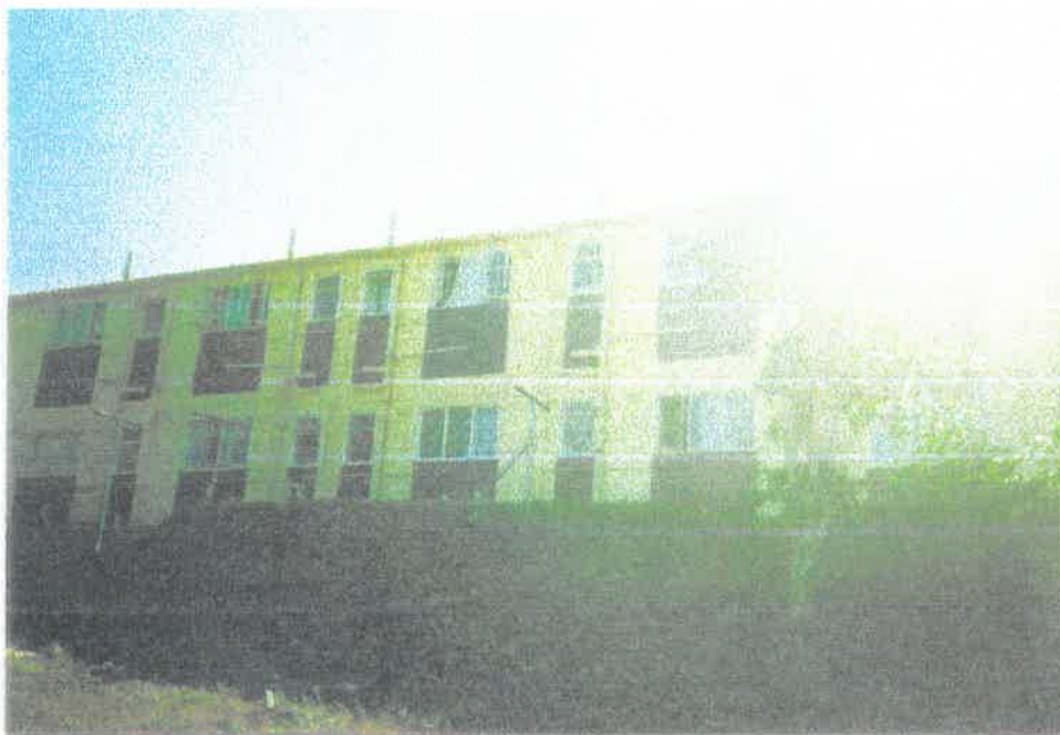
7b. Rear view of block of flats with only one entrance per unit.
