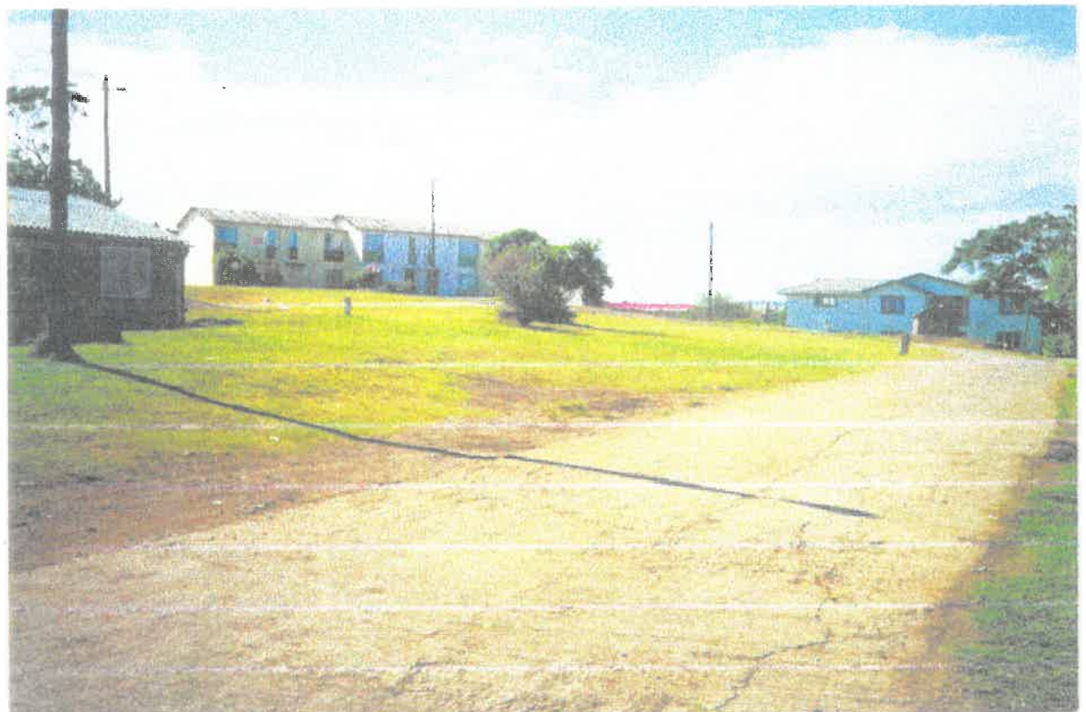
13. Haphazard construction of roads.
