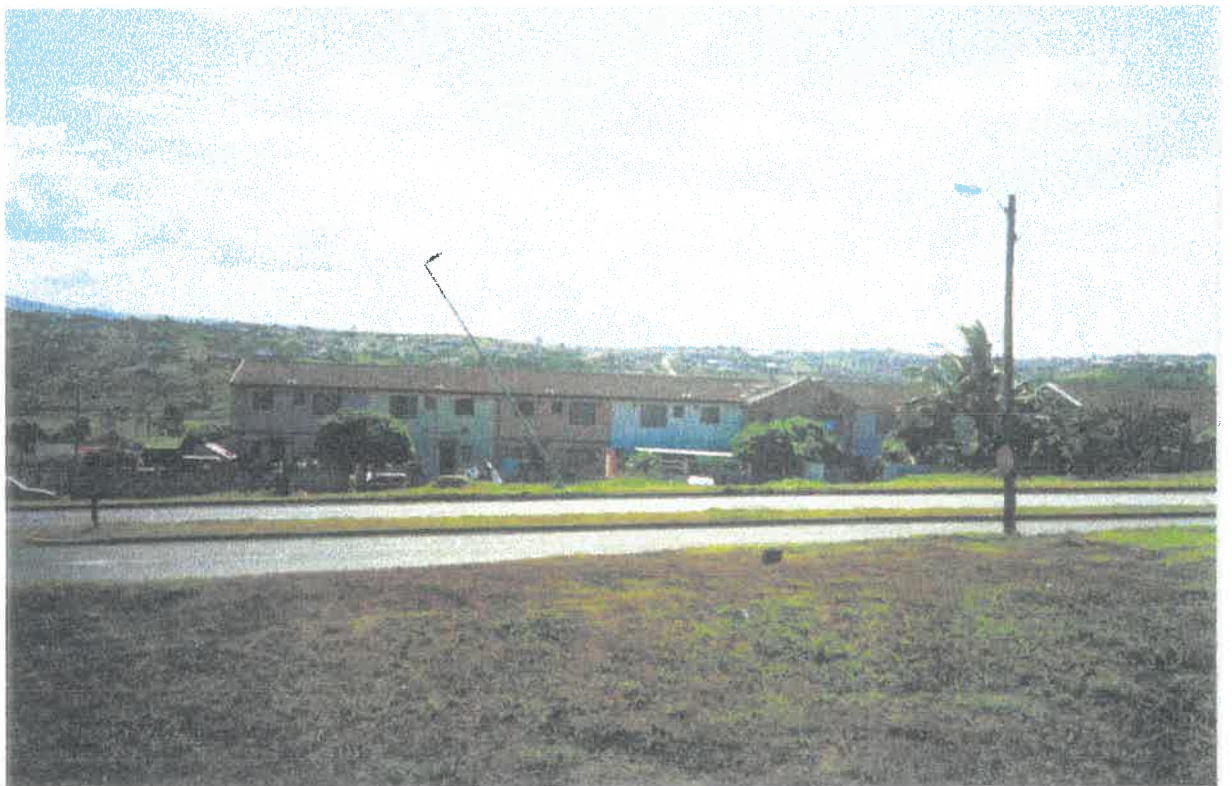
2. Terraced (tiled roof) houses.
