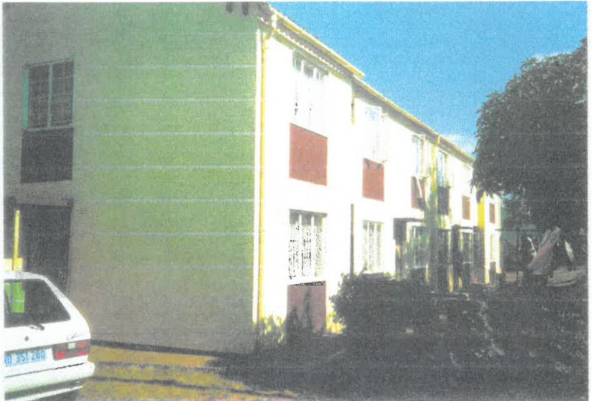
7a. Front view of block of flats with only one entrance per unit.
