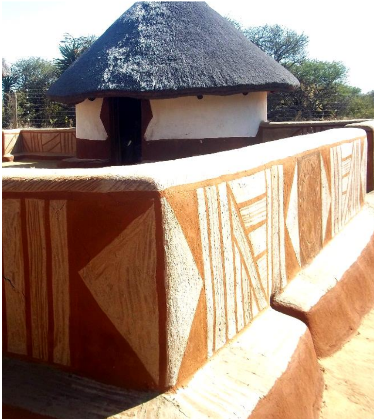
Figure 6: Traditional Sotho-Tswana house and wall painting. Bakoni Malapa Northern Sotho Open-Air Museum. Photograph by M.F. Motsamayi, 2014.
