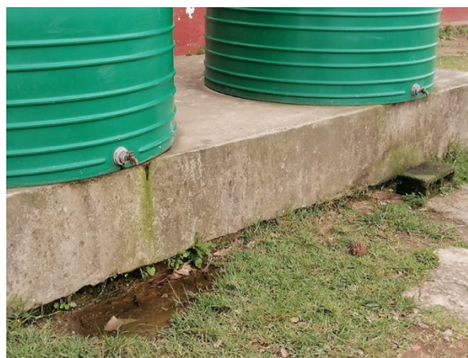
Figure 4.4: Kaniso's photovoice: "Unsafe spaces: water shortage"
