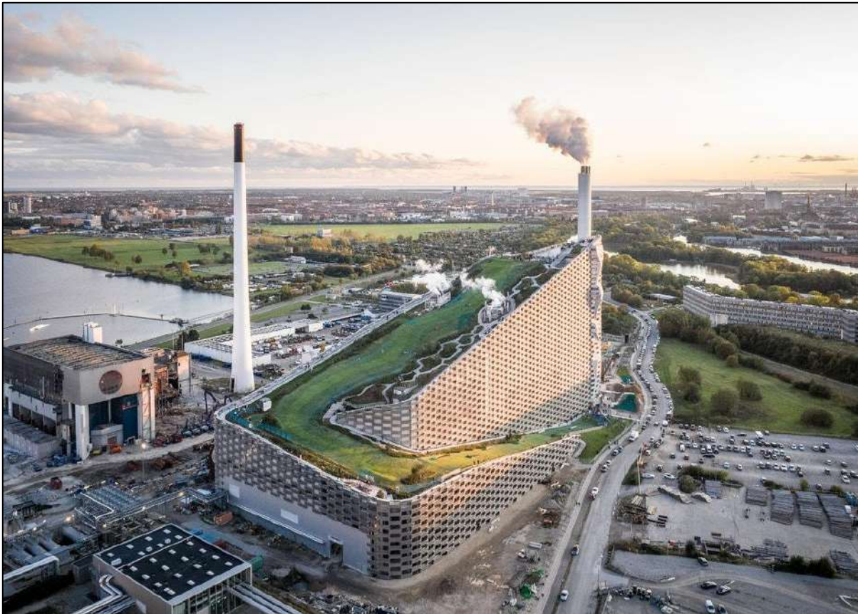
Figure 5.8: The Copenhill, also known as Amager Bakke, in Copenhagen Netherlands set within the surrounding industrial context.
