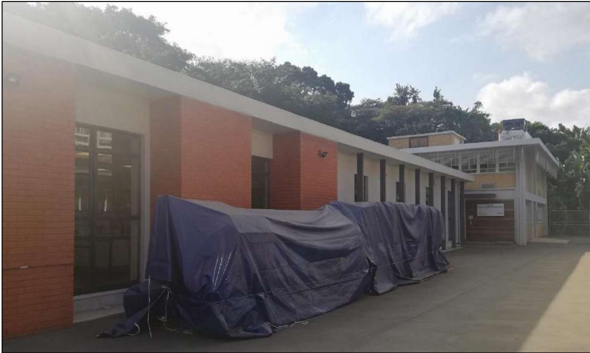
Figure 6.2: The Biorefinery Industry Development Facility set within the CSIR in Durban.
