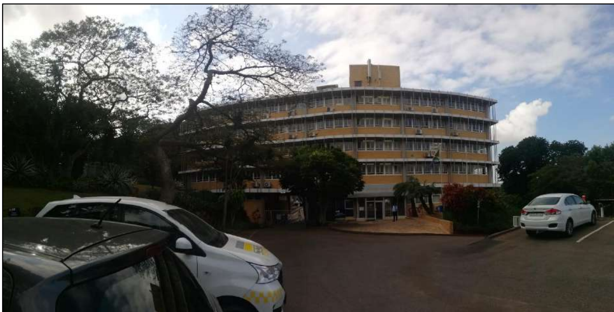
Figure 6.1: The Council for Scientific and Industrial Research main building set within the surrounding context of the University of KwaZulu-Natal, Durban
