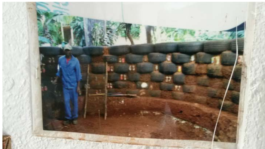
Figure 45. Picture taken showing the construction of the earthship (Author, 2014).
