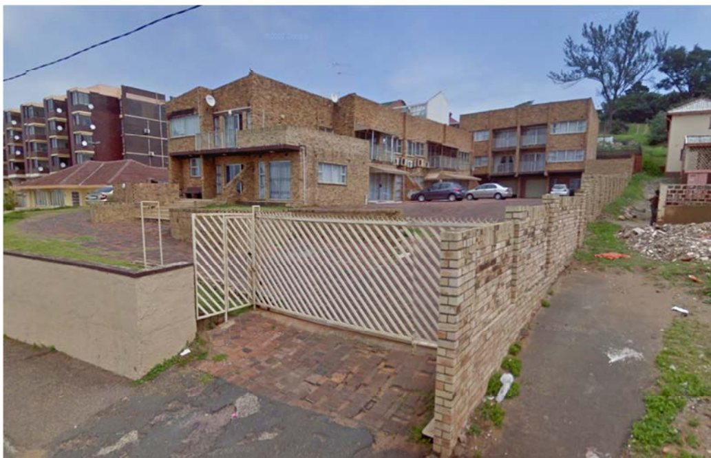
Figure 30. Street view of original property (Google Earth, 2013).
