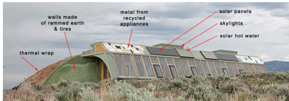
Figure 2. Typical earthship (Lejuwaan, 2012).
