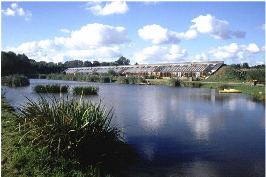
Figure 18. View of the Hockerton Housing Development (Alasdair Morrison and Partners).
