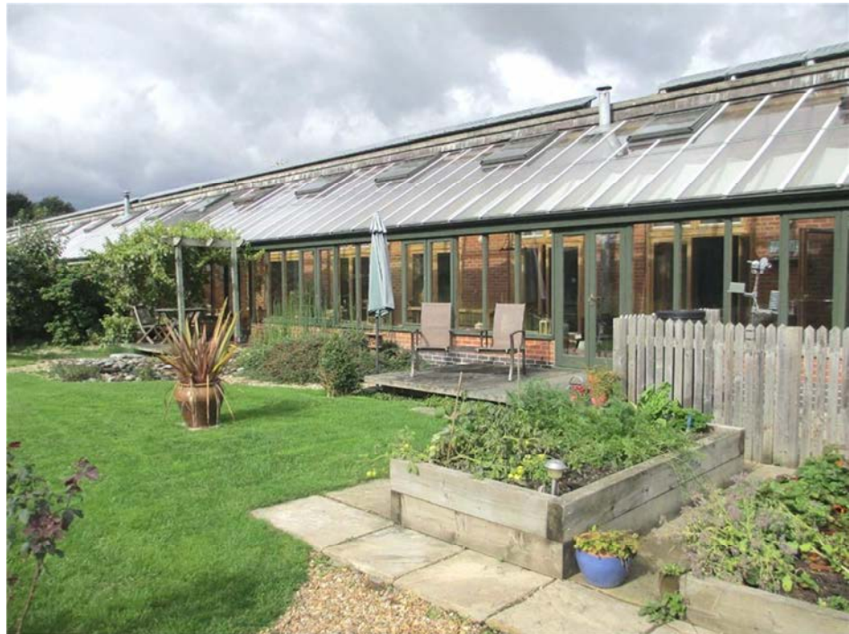
Figure 20. Front of building showing conservatory, private garden and photovoltaic array on the roof (Alasdair Morrison and Partners).
