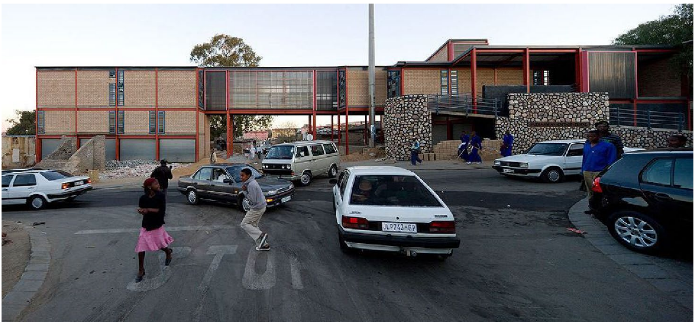
Figure 44: Large sections of locally created brick infill were incorporated into the building's northern façade by the local community
