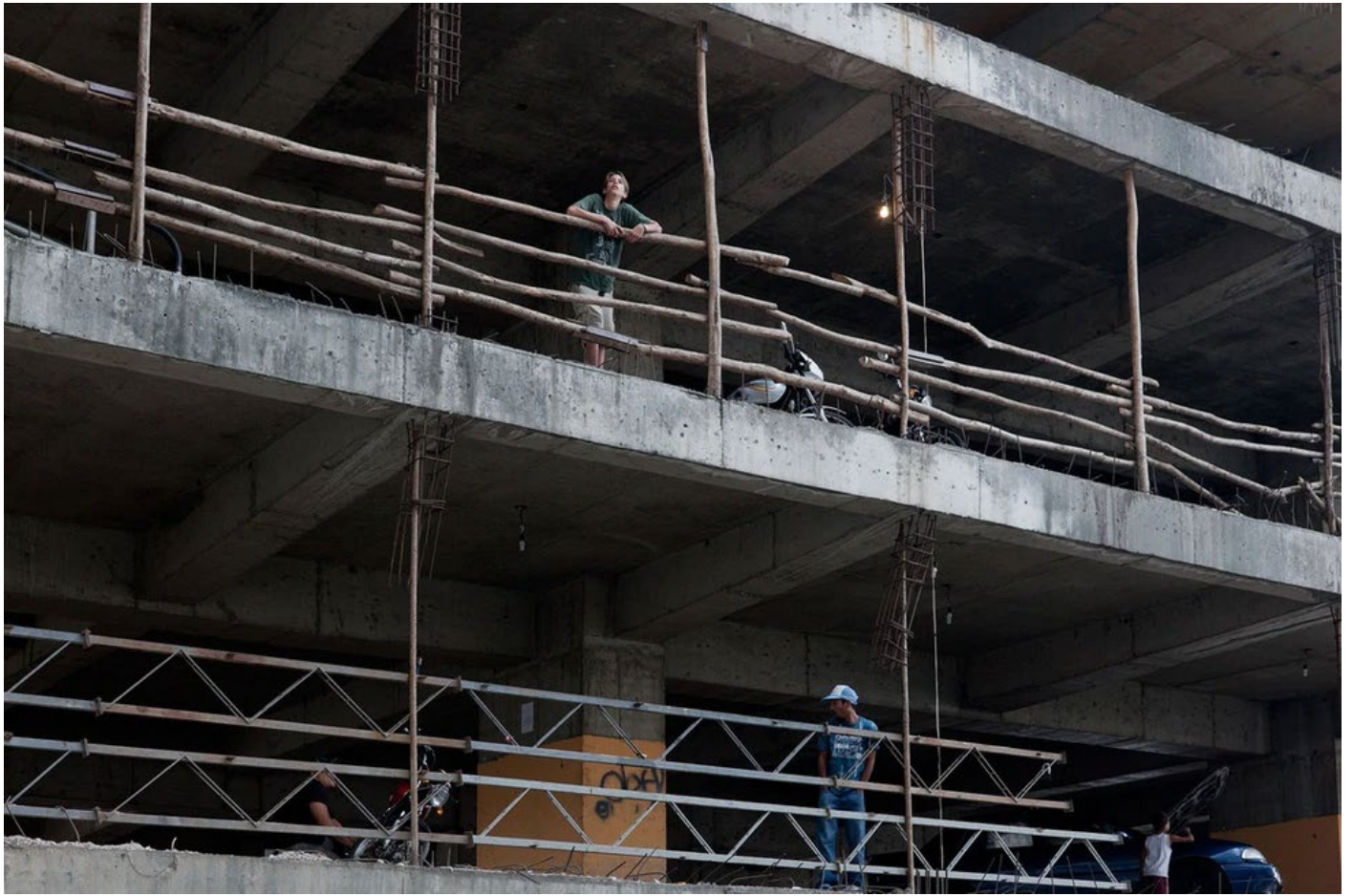
Figure 55: Residents created timber balustrades with timber logs found locally. Source: Afasiarchzine (2012). 21 April 2023
