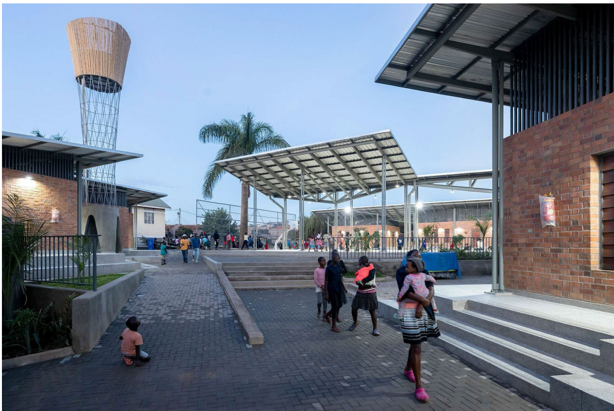
Figure 36: A view of the site indicating the different platform levels, water tower, butterfly roof, and buildings Source: Design boom (2022). 12 April 2023
