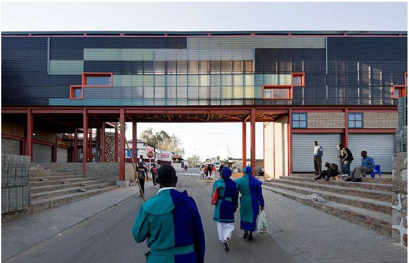
Figure 45: The steel frame construction of the main exhibition space is filled with contrasting brickwork, polycarbonate sheeting, and other forms of corrugated metal.
