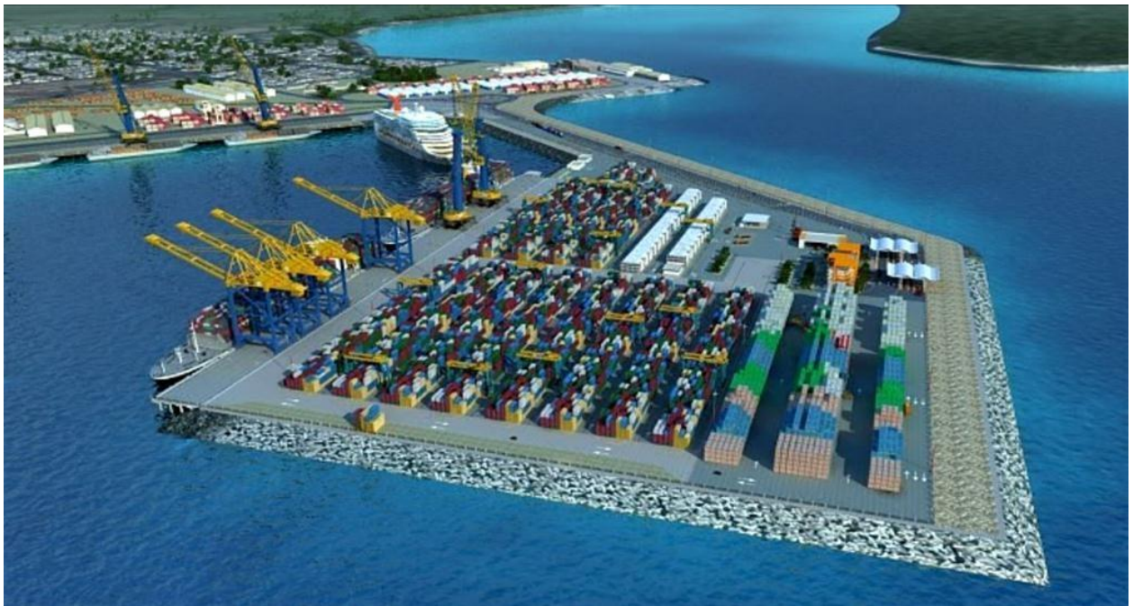
Figure 1.3 New Terminal after Completion
